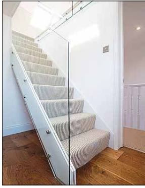
White, wood and glass: a clear balustrade maximises light in the Clapham flat
